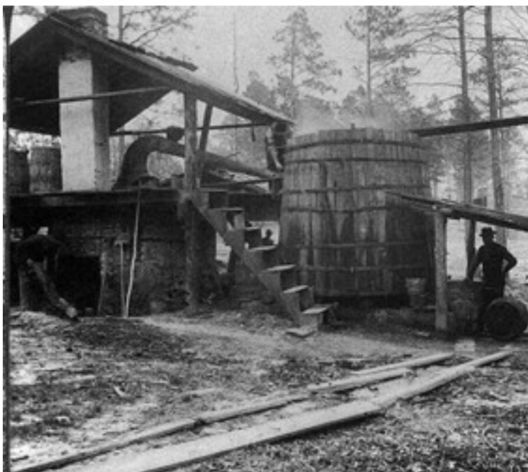
Distilling turpentine from the crude resin in the pine forests of North Carolina 1903 ( DaysGoneBy )
